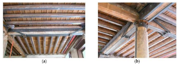
Figure 1. Retrofitting with steel-wood composite beams (a) steel plates along beams; (b) steel profiles at column joints [5]
