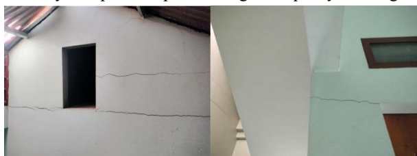
Figure 1. Cracks in residential houses caused by ground vibrations from blasting during road construction in Yen Bai Province
