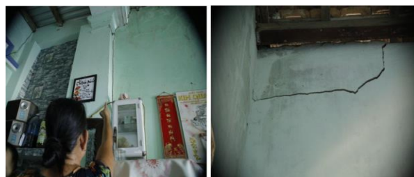
Figure 2. Cracks in residential buildings due to vibrations from pile driving for the embankment construction in Quang Nam Province
