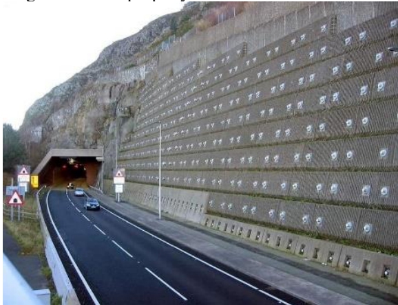
Figure 1. Roadbed reinforcement anchor
