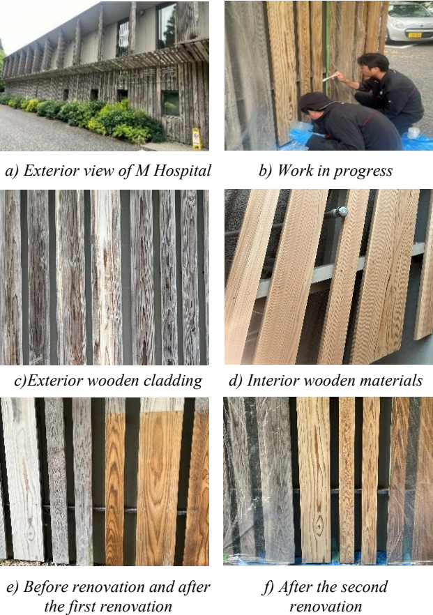
Figure 7. Renovation of the Facility Using a High-Elongation Acrylic-Silicone Transparent Protective Coating
