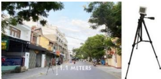
Figure 1. Illustrate the arrangement of monitoring equipment at the 4 measurement positions
