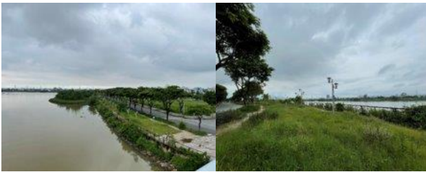
Figure 9. Current state of Thang Long road in Danang
