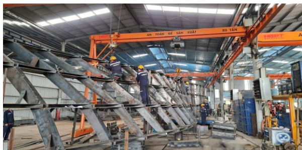
Figure 18. Construction image of stainless steel structure - curved dome from Ha Giang Phuoc Tuong Mechanical Joint Stock Company in Danang city
