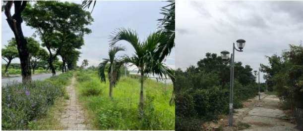
Figure 10. Current state of Thang Long road's infrastructure in Danang
