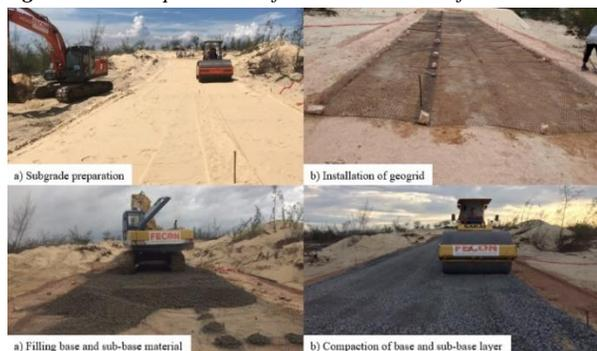
Figure 6. Construction process of trial test in Quang Binh B&T windfarm project
