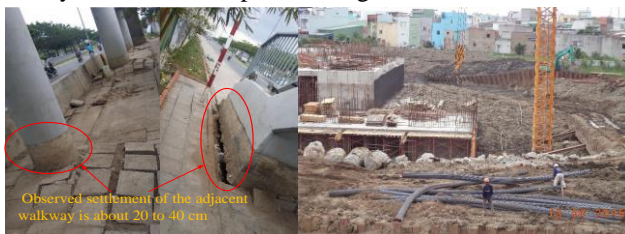
Figure 14. Settlement of the soil affects the neighboring structures of the actual construction project in District 8, Ho Chi Minh City
