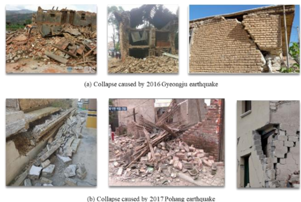
Figure 1. URM walls collapsed during earthquakes occurred in South Korea
