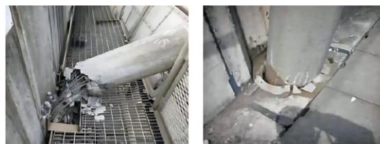
a) Example of breakage b) Example of inclination
