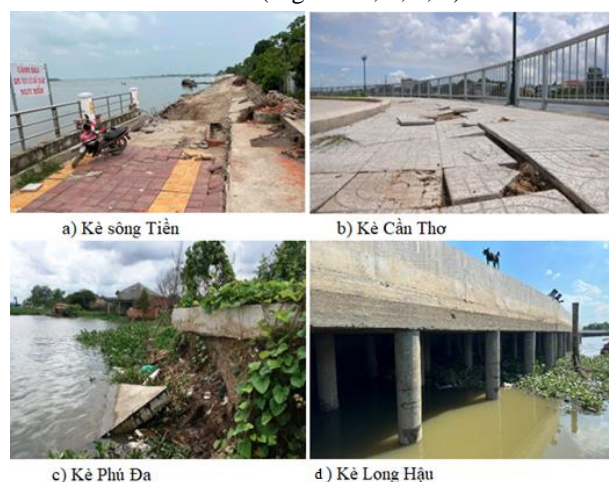
Figure 1. Some typical images of embankment incidents
