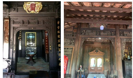
Figure 5. Forms of family doors - "Vong door" decorated in square or rectangular shapes, according to the lean-to of the house (Source: the author)
