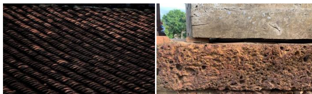
Figure 6. Construction materials: yin-yang roof tiles and original wooden and laterite foundation (Source: the author)
