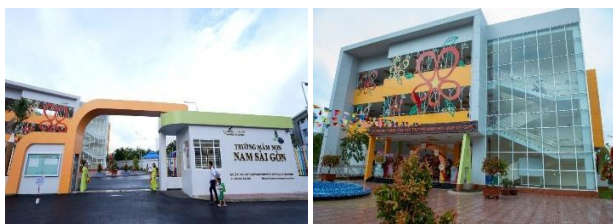
Figure 4. Saigon South Kindergarten, District 7 - Source: [4]
